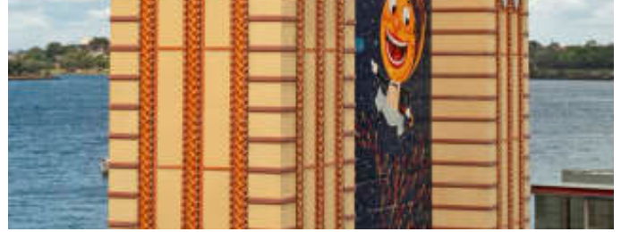
Luna Park’s entrance pays homage to New York’s Chrysler Building. PETER SHERIDAN
